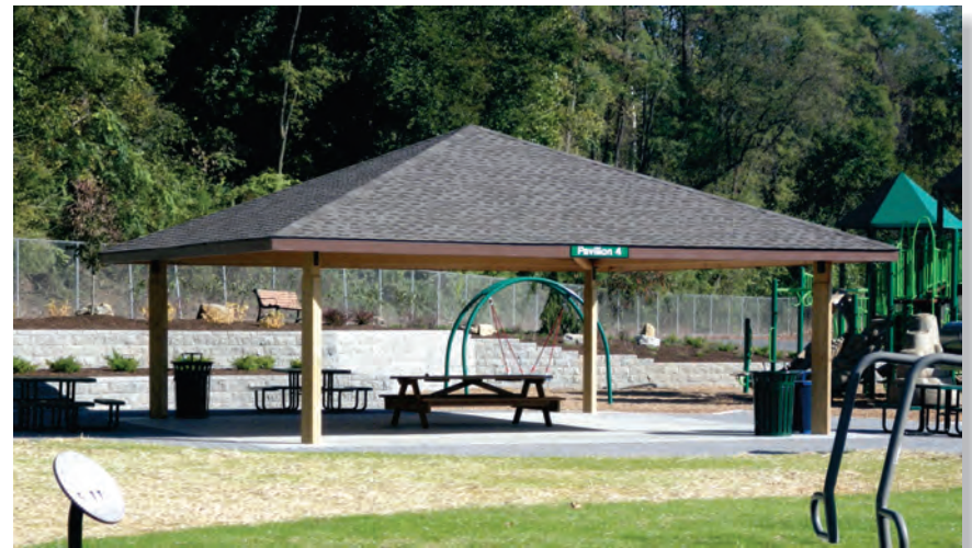
Pavilion 4 New Pavilion (#4) - 40/50 People $15 per Hour
