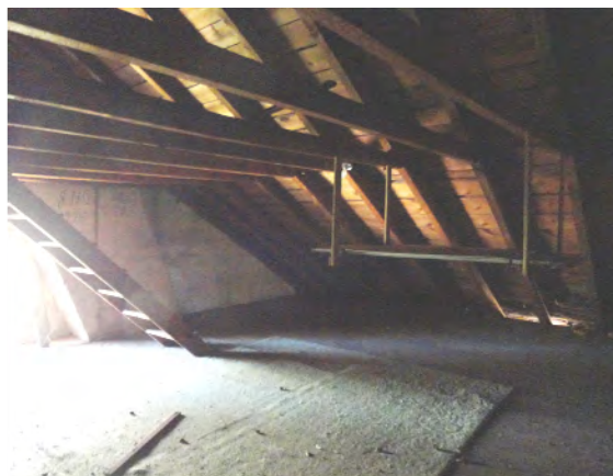
Attic area once used as a pigeon roost.
