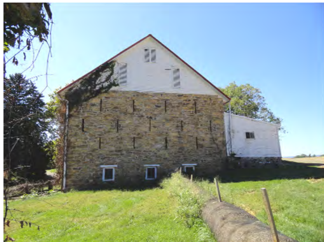
“Stone End” with typical venting
