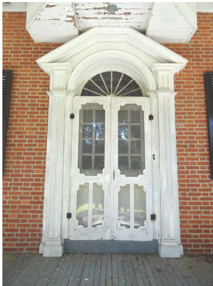
Main Entry Door to Mansion House
