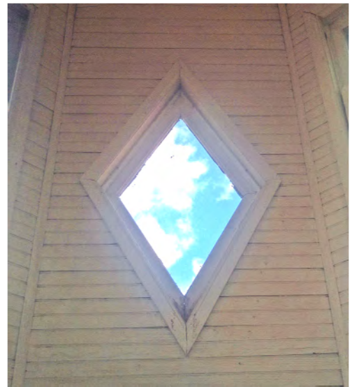
View through the Roof Monitor
