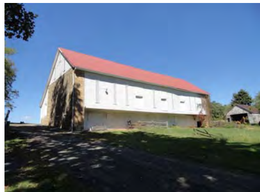
The Stone End Bank Barn
