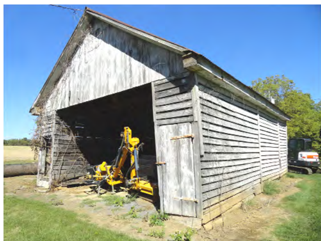
Corn Crib/Wagon Shed near the Barn
